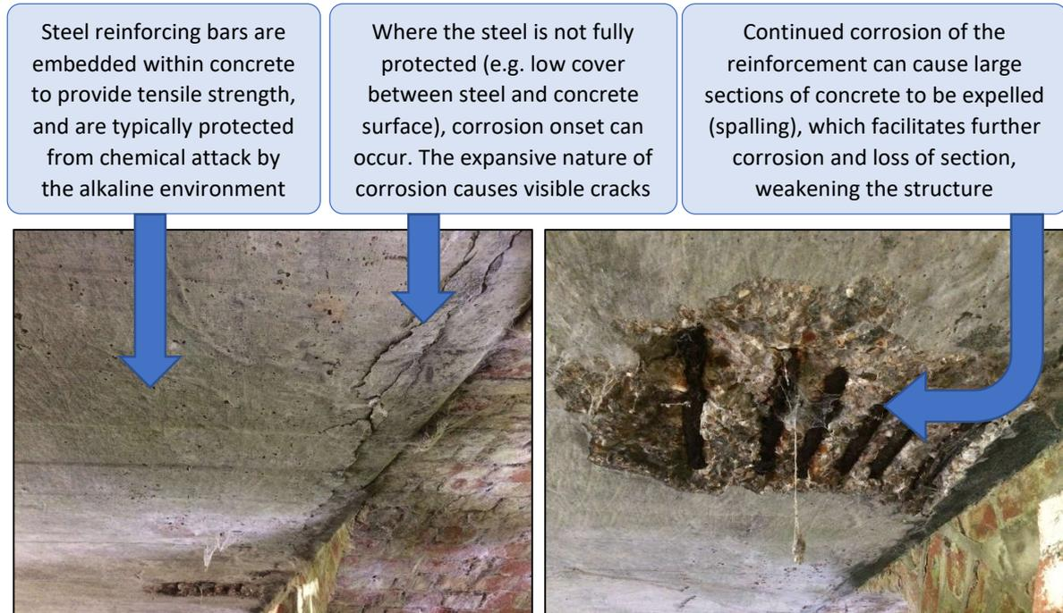
Figure 1 – Reinforcement corrosion-induced cracking and concrete spalling in a normally-reinforced concrete deck slab
